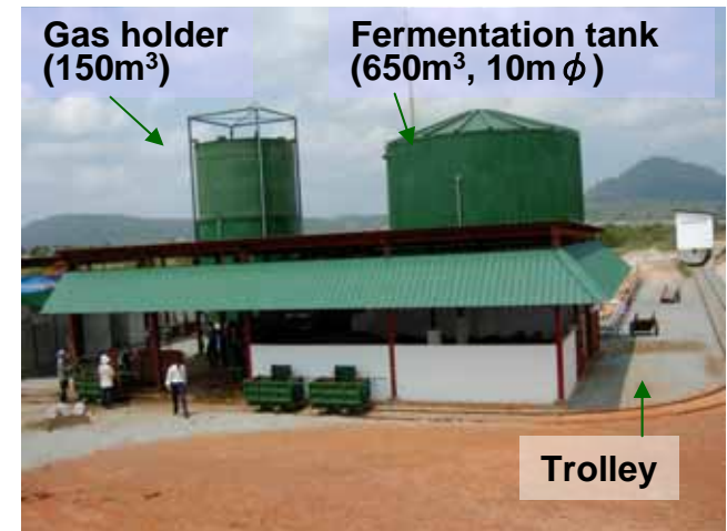
Biogas fermentation tank
