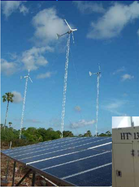
PV-Panel, total cap 35 KWh, combined with wind turbin @ 10 kW
